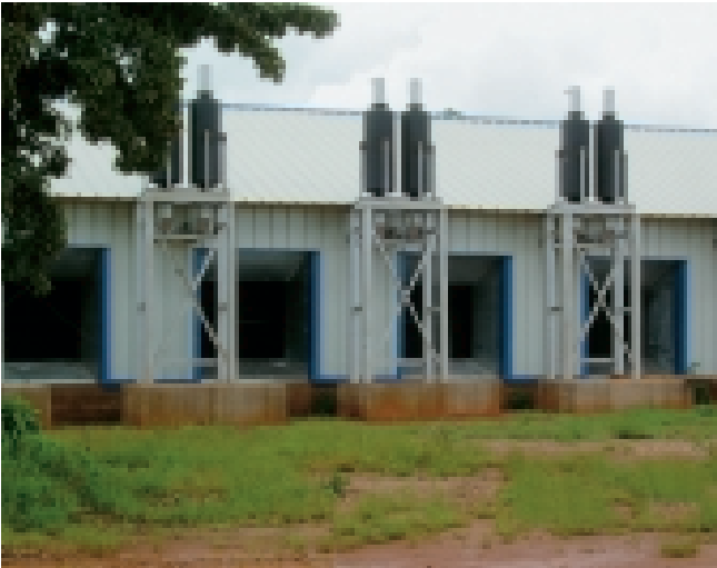
Installation of eight C1400 D5 generator sets
