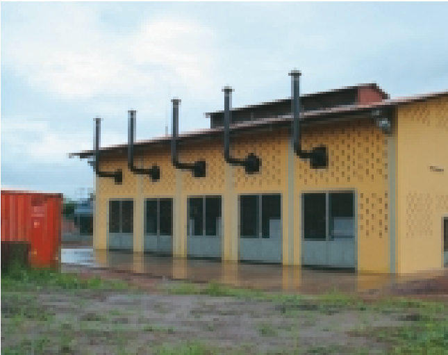
Installation of five C825 D5 generator sets
